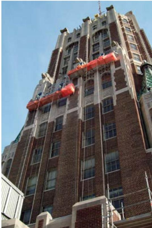
Fig. 7: Swing staging with larger work platforms and ability to capture debris
